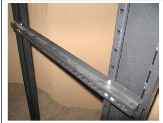
Please attach 'Cage nuts' to horizontal profiles before bolting to the frame using holes 4 & 5 (600mmX600mm, 600mX800mm Cabinets only)
