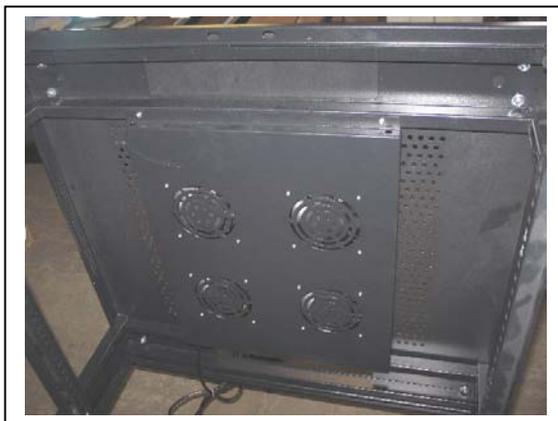
Carefully attached the supplied 'Fan Tray' to the top of the inner surface of the installed perforated roof.
