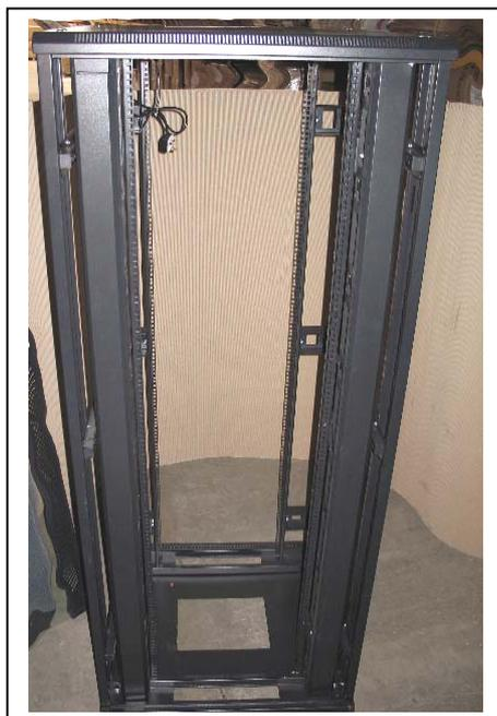
Carefully install the vertical cable management cable trays (x2 supplied)
